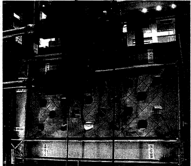
Figure 6: Damage to panel and boundary frame (Specimen P: End-of-test, \gamma = 3.0\% \approx 10\delta_y )
